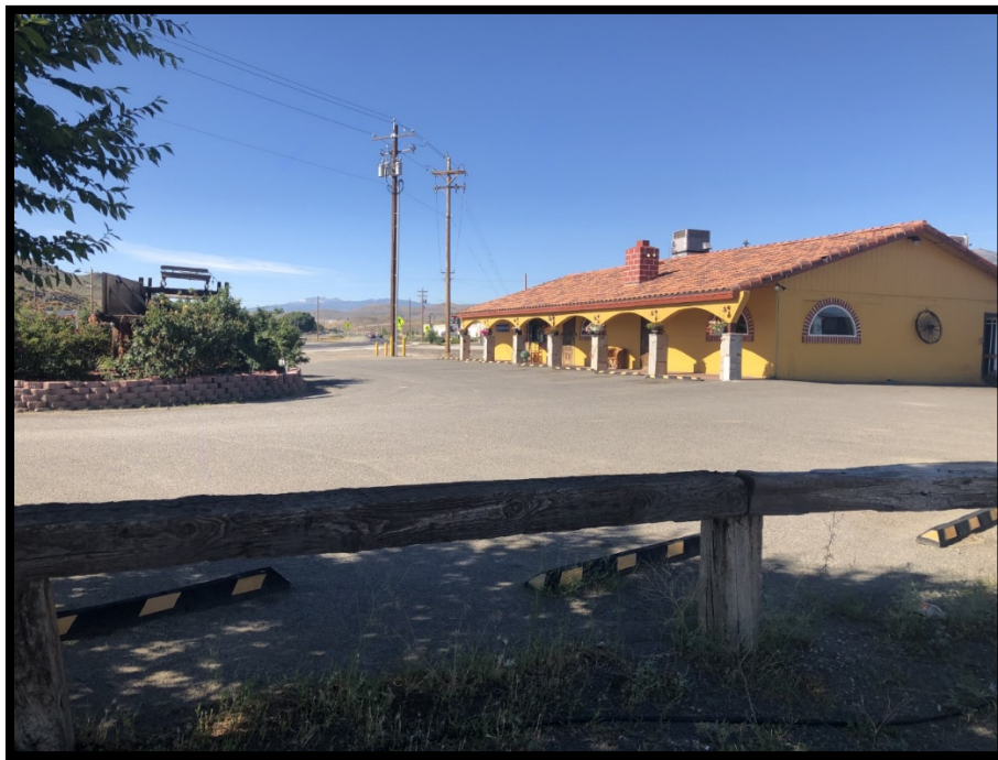
Photo 3: Restaurant and parking area located on Parcel 3.
